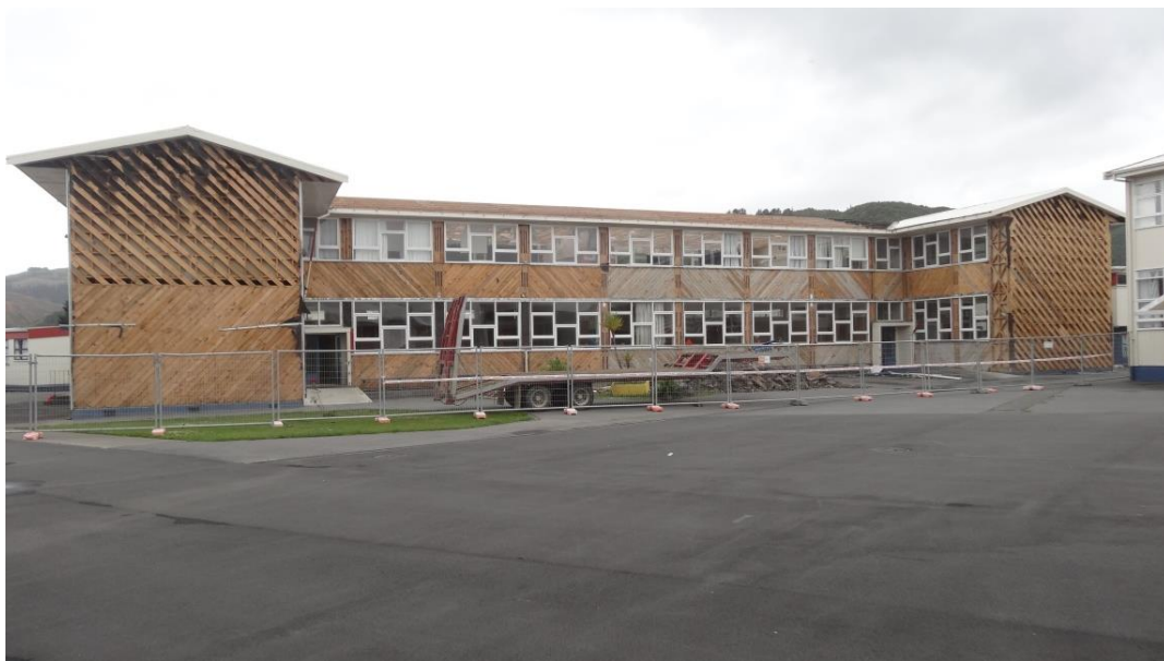
Figure 1: Two-storey Nelson Block with Sarking Exposed Prior to Demolition
