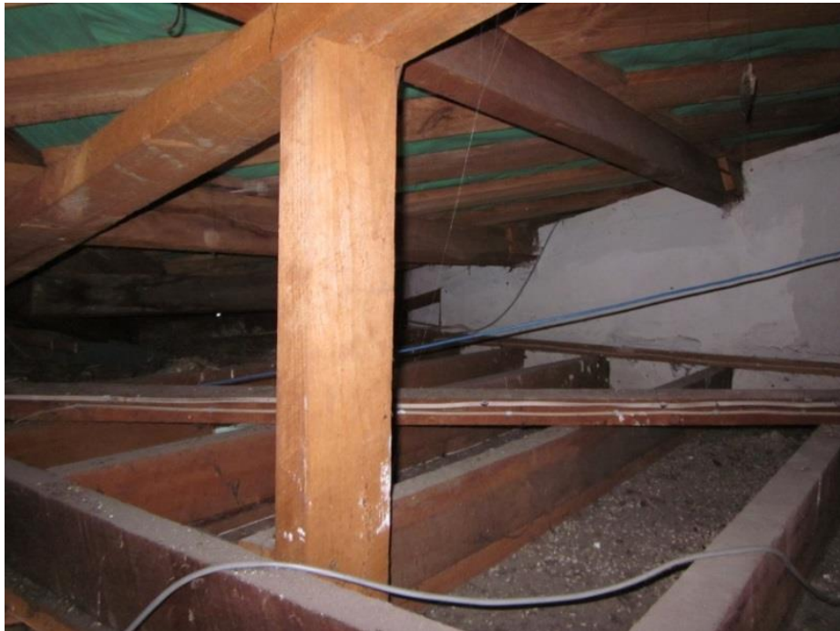
Figure 3: Inspected Roof Framing in End Portion of the 'H' Section
