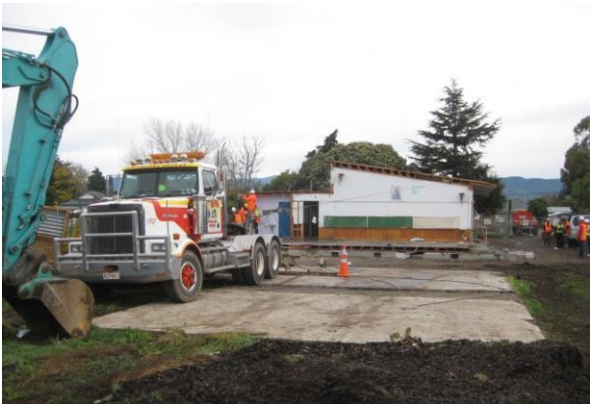
Figure 3. View of the Avalon block during testing
