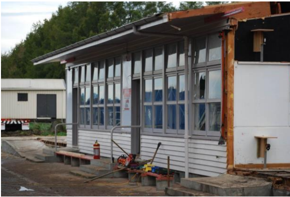
Figure 4. Building at end of longitudinal test
