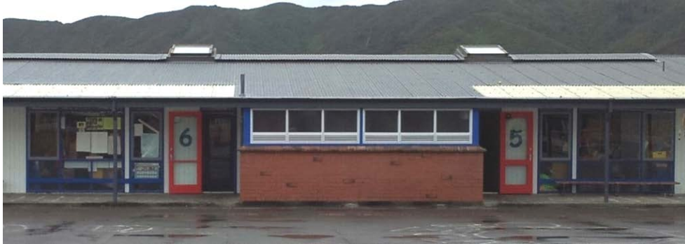
Front view of typical 2-classroom Formula block
